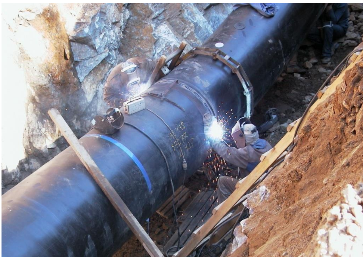
Welding of a high-pressure gas pipeline
