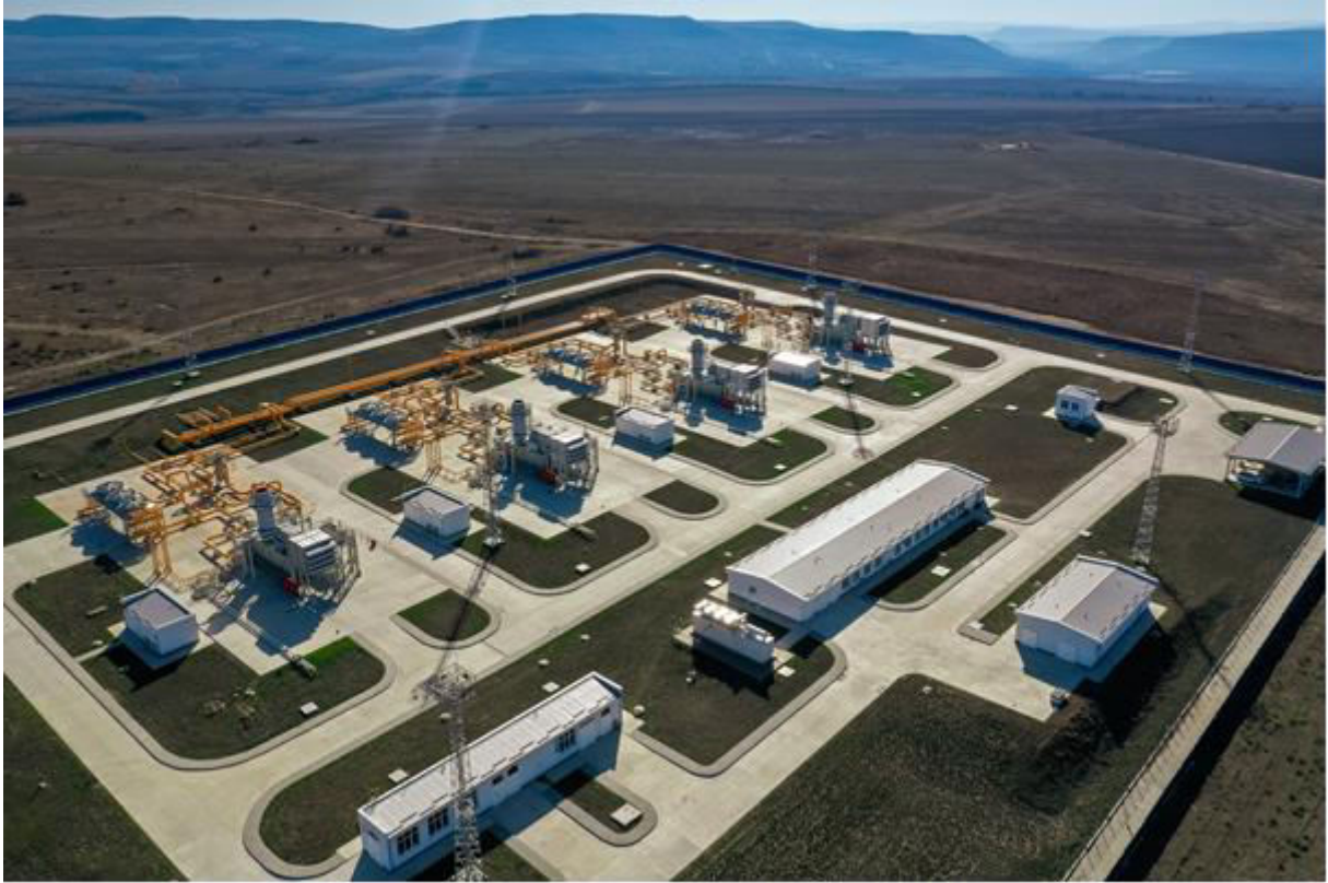
Compressor Station Nova Provadia
